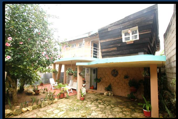
After: New Home in Fermathe being refurbished
